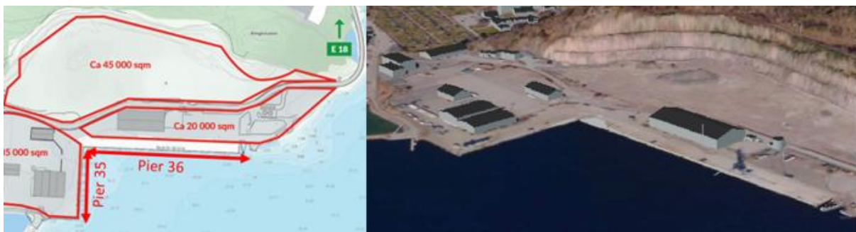
Figure 13: Port infrastructure foreseen for OW O&M hub
